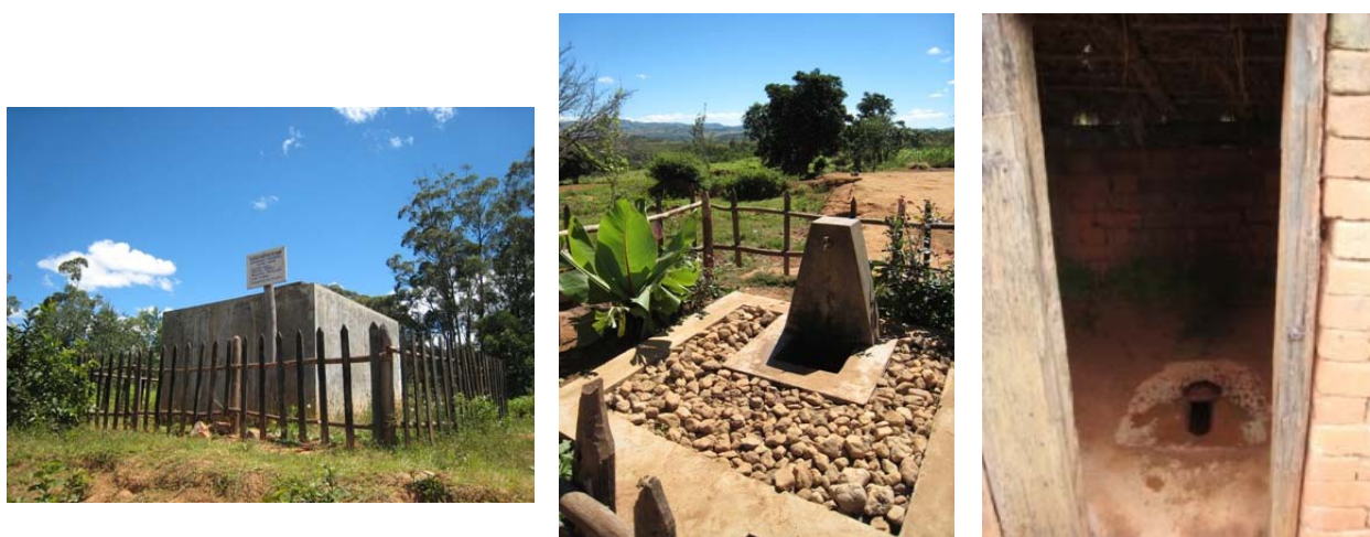
Figure II.1: Water tank, tap stand and pit latrine installed in Ampila by WaterAid and SAF/FJKM
